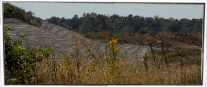
Meredyth Mine near Haleyville, AL pollutes Bear Creek, a tributary of the Tennessee River.
