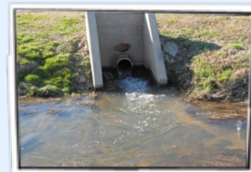
Discharge pipe from Ardmore WWTP
