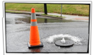
This photo shows untreated sewage overflowing from a manhole cover.
